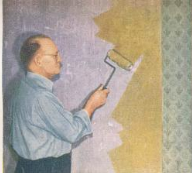
Left, new type of paste now on market is applied to wall instead of paper. Paper is unrolled on wall, eliminating cutting
